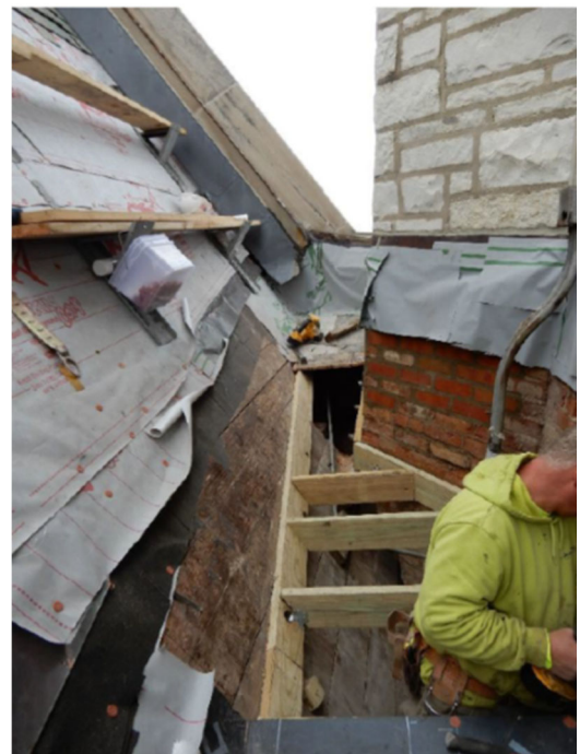
rebuilding the cricket assembly
