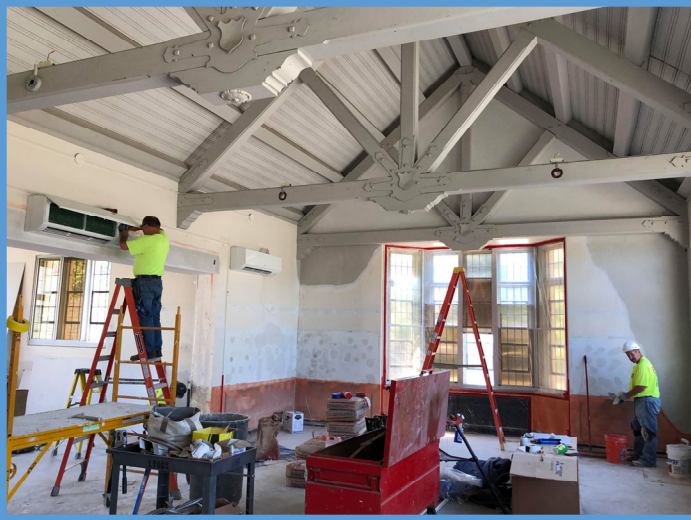
Former kindergarten room, now the new Holy Name Room.
