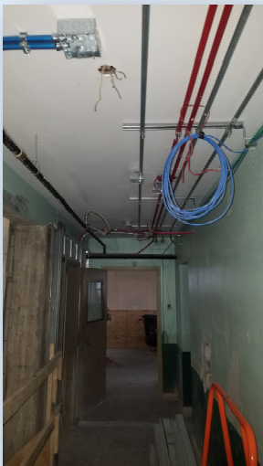
Hallway in the Basement
